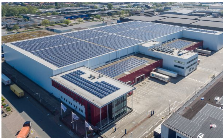
Figure II.3 : Frigomundo Coldstore in THE NETHERLANDS, Zouterwoude [12]
