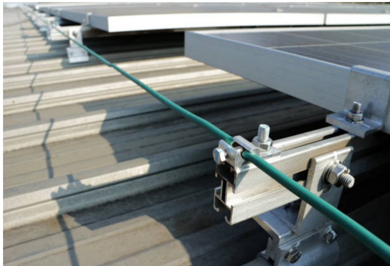
Figure I.16 : Grounding system on a roof [18]
