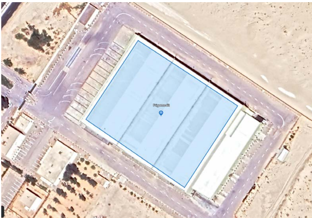
Figure IV.2: Upper view on Frigomedit El-oued
