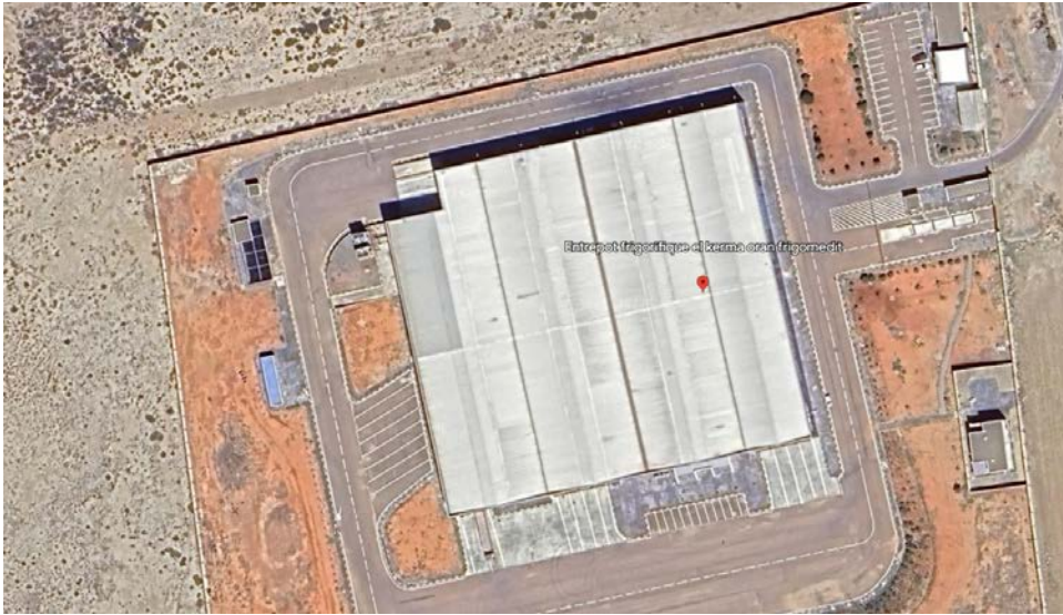
Figure IV.17 : Unit of Frigomedit at El karma Oran
