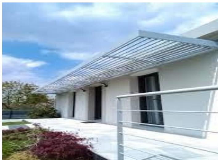
Figure III-32: Brise-soleil à lames horizontales [29]
