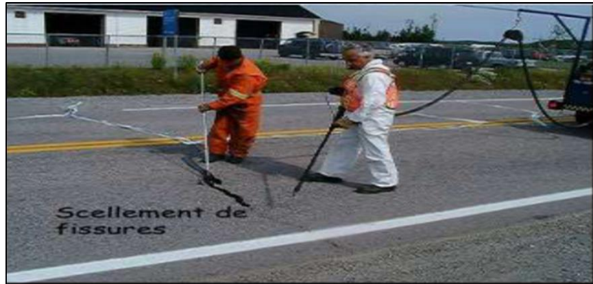
Figure I.18: Scellement de fissures[3]
