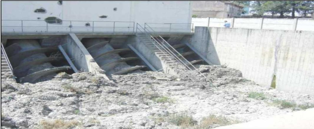
**Figure IV.42:Etat de station de relevage SRG 2**
