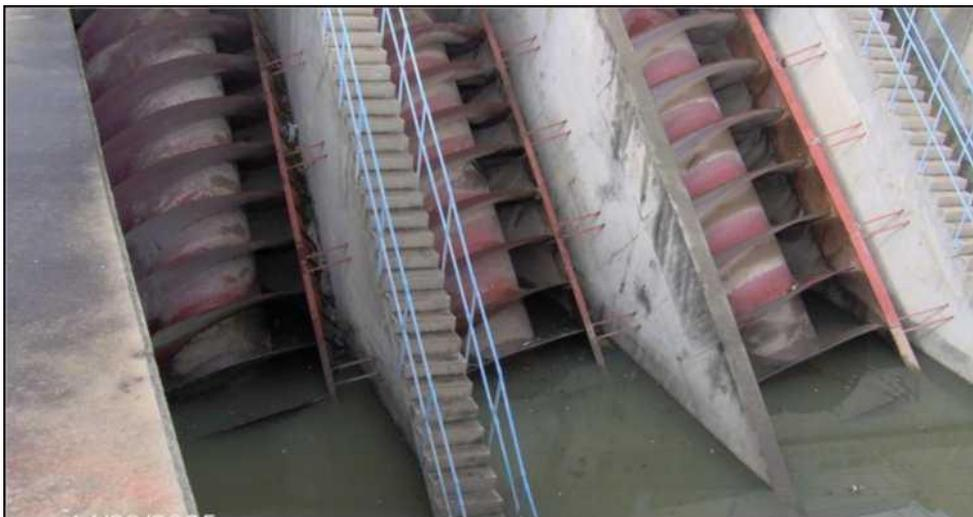
Figure IV.2: Poste de relevage N°1(PR1)
