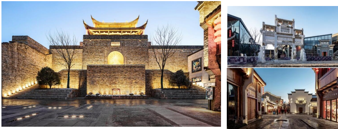
Figure 21 photo du projet de wuhu. source: https://www.architecturepressrelease.com/winner-wuhu-old-city-phase-i-pt-architecture-design-shenzhen-co-ltd/
