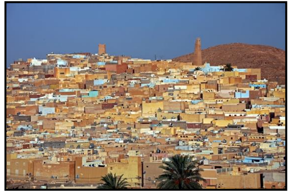
Figure 96 : photo de ksar beni isguen. Source: OPVM
