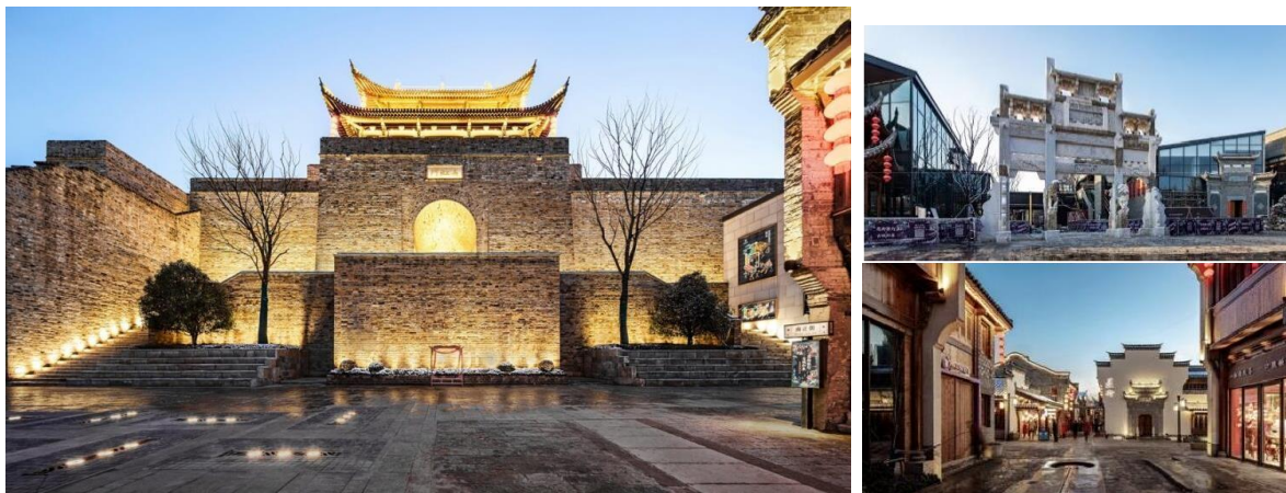
Figure 21 photo du projet de wuhu. source: https://www.architecturepressrelease.com/winner-wuhu-old-city-phase-i-pt-architecture-design-shenzhen-co-ltd/
