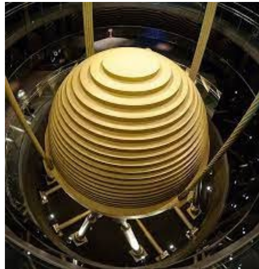
Figure I.2 : TMD Pendulum of Taipei 101.
