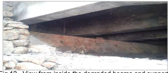
Fig.12 - View from inside the degraded beams and support.
