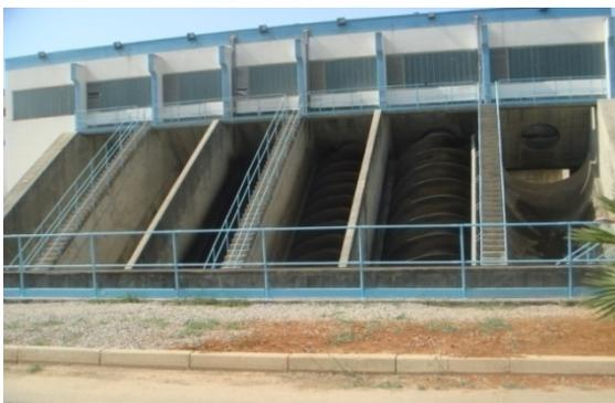
Figure III.8: Poste de relevage PR1
