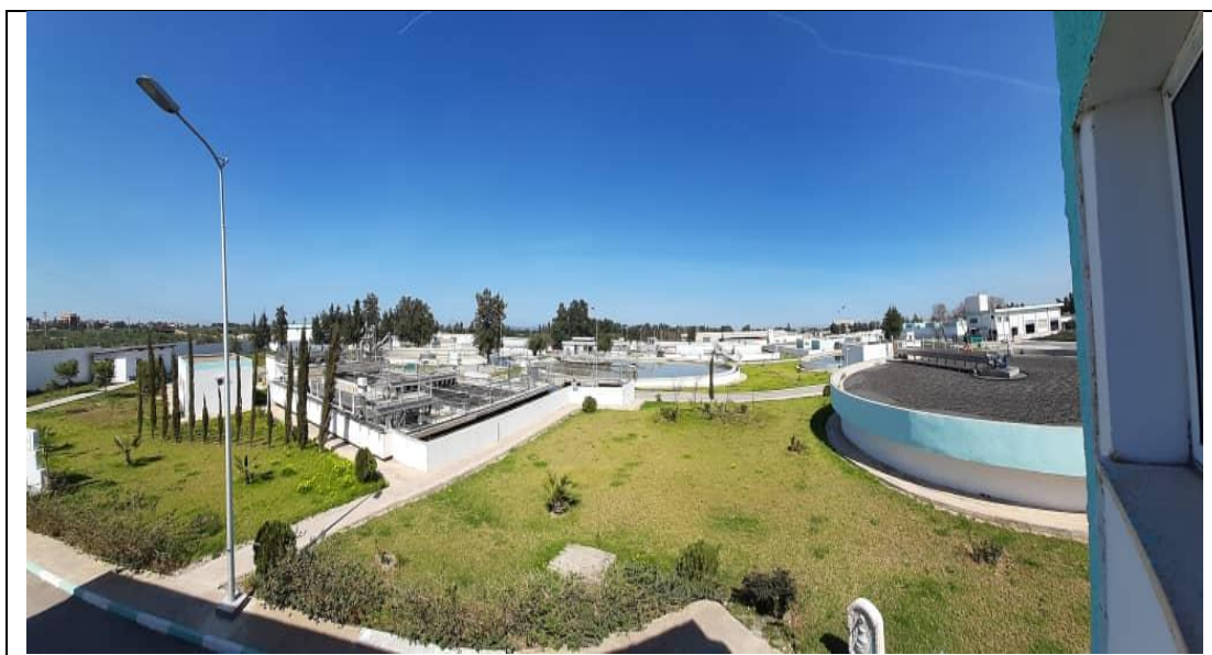
Figure 1 : Station d'épuration de Béni Mered (Photo originale)
