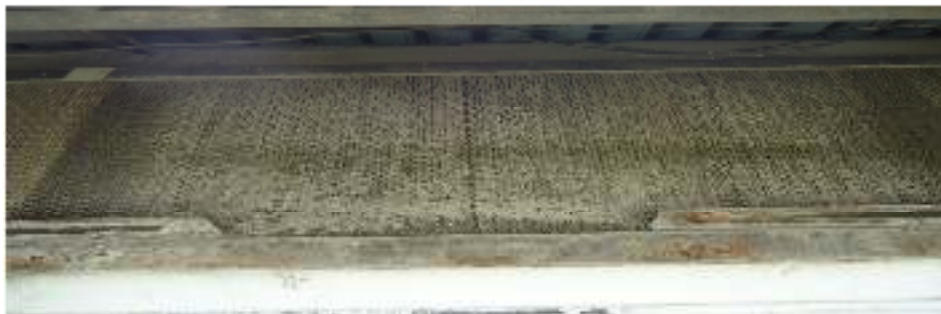
Figure 9: Les pad-cooling
