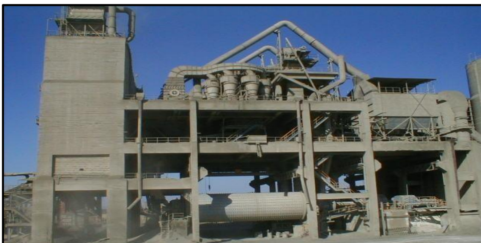
Figure 1-10 : Zone ciment SCMI
