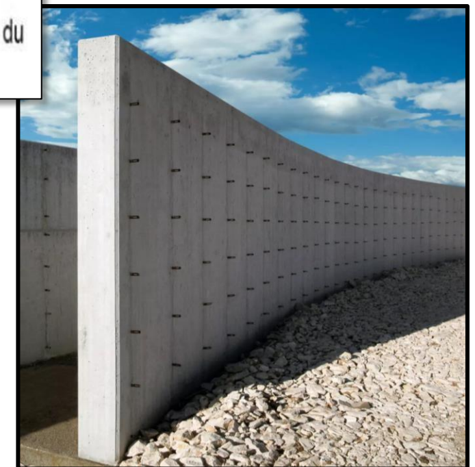
Figure 50.voiles de contreventements.
