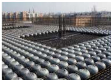
Figure 126 : plancher cobiax
