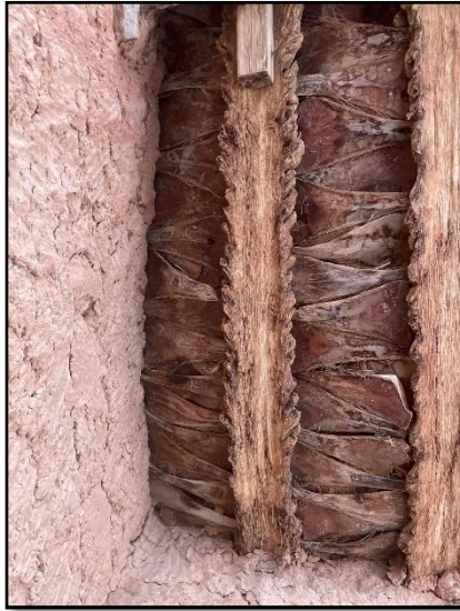
Figure 3: Technique de construction
