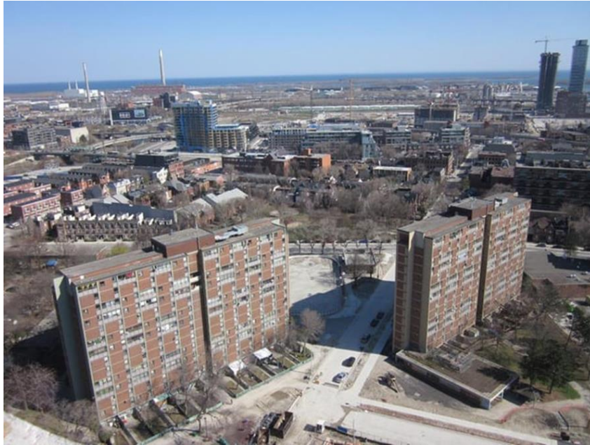
Figure 08. Peter Dickinson towers at Shuter and Dundas, demolished in 2014.
