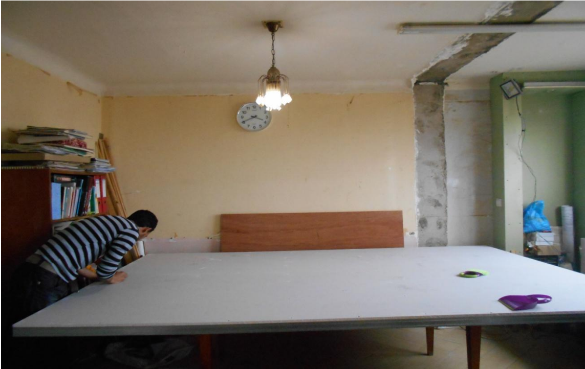
Figure 4.6. Construction de la table.
