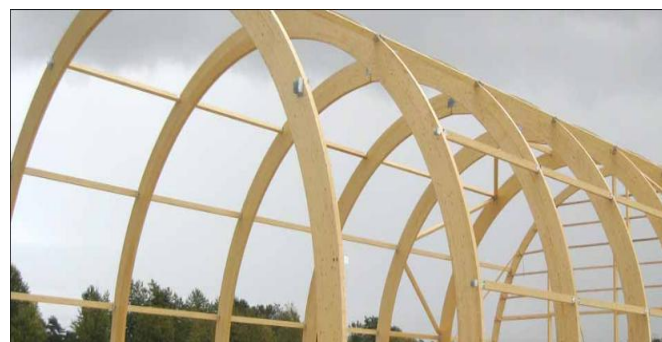
Figure 83: Charpente en lamellé collé, google image
