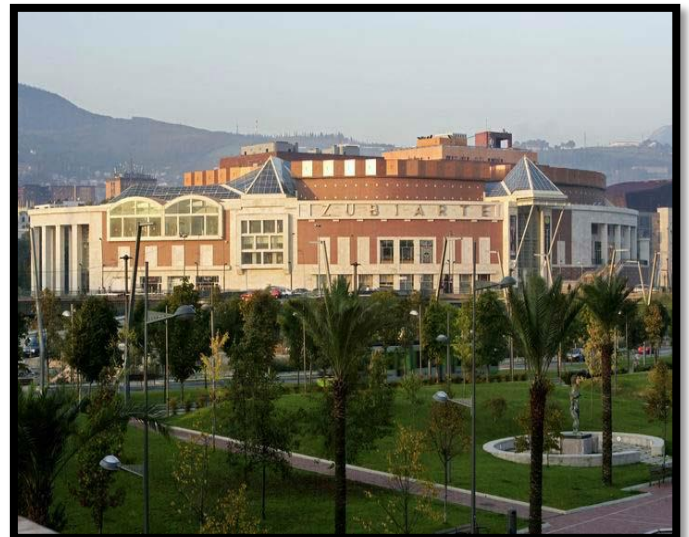
Shopping centre Source Bilbao Ria 2000
