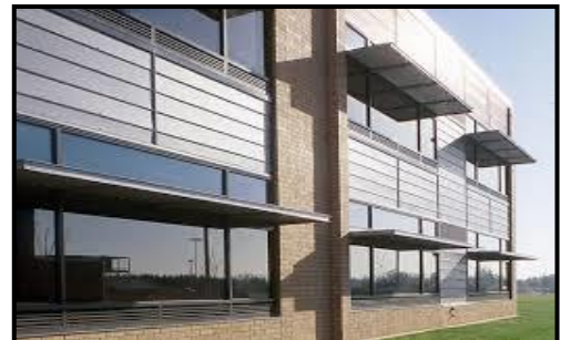
Figure 115: le système light shelf. Source:gordon-inc 2014.
