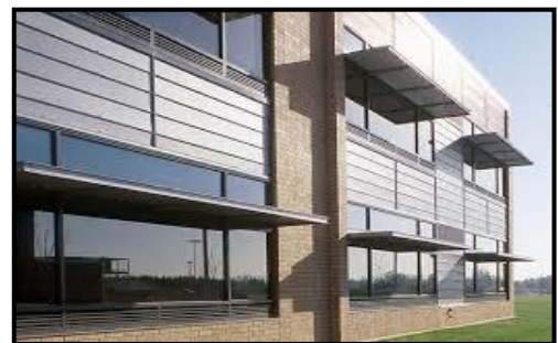
Figure 115: le système light shelf. Source:gordon-inc 2014.
