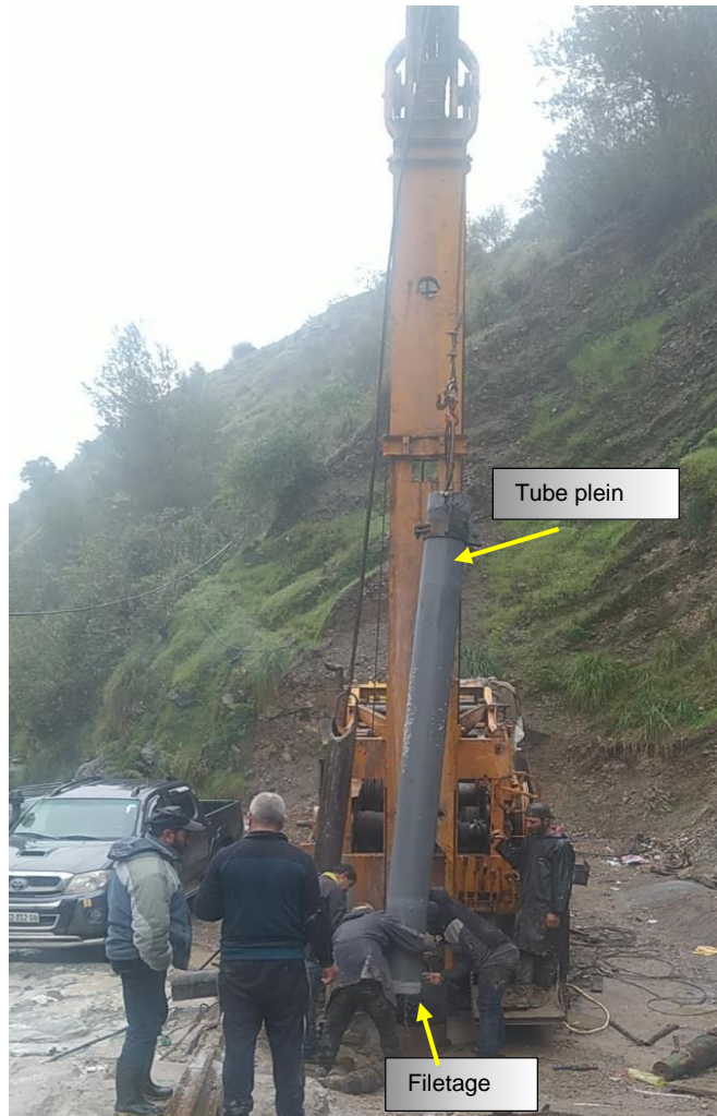
Figure III.16 : descente de tubage
