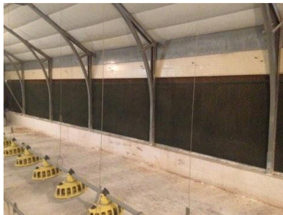
Figure 7: Pad-cooling
