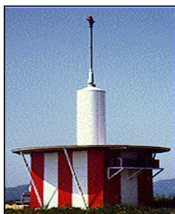
Figure III. 9. Station CVOR/DME
