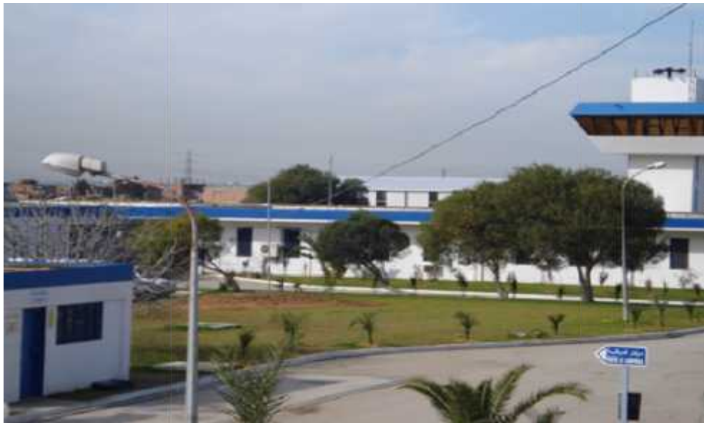
Figure 2 : station de traitement BOUDOUAOU(photo originale, 2015)
