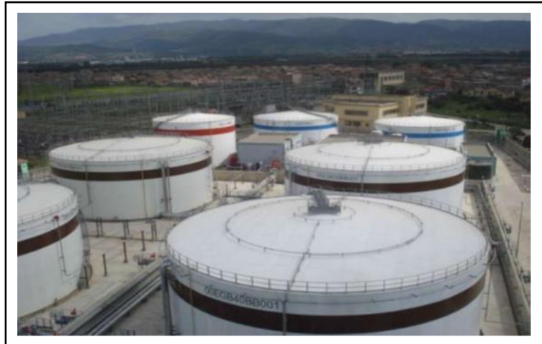
Figure 1.6 Station de carburant.
