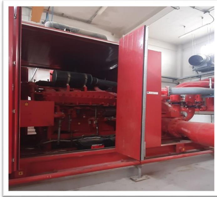
Figure 2.4 pompe diesel.
