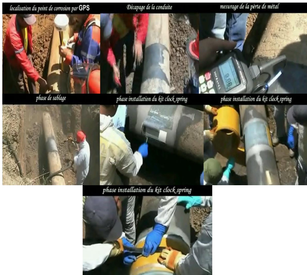
Figure I.10: Installation de Clock Spring [12]
