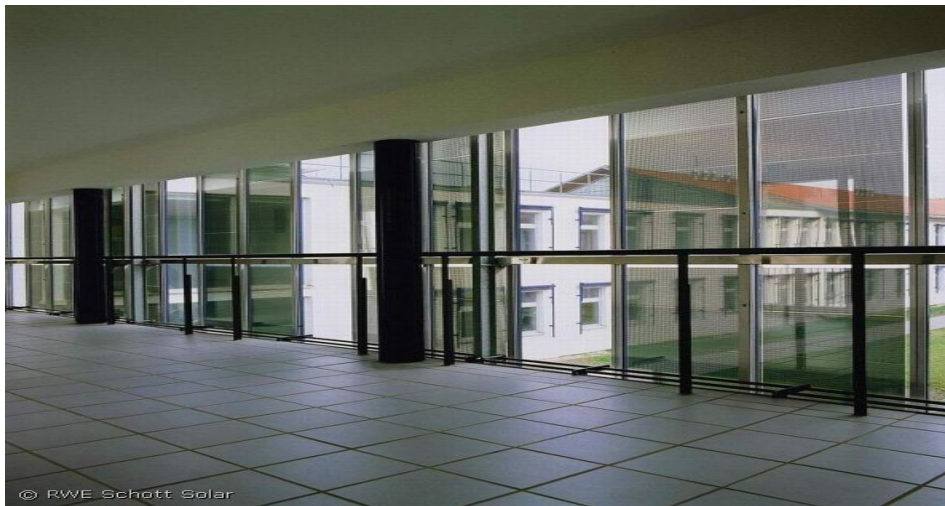
Figure IV.6 : modules transparents
