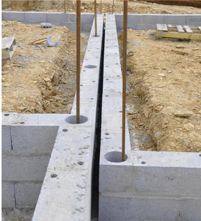
*Figure XII.2: Joint de rupture.*
