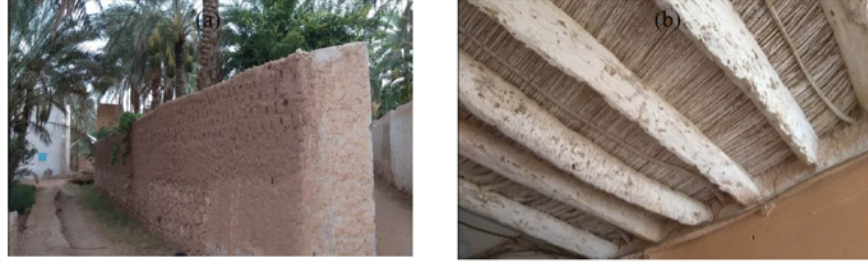
Figure 2.12: (a) Earthen wall in the palm grove house of Béni Isguen; (b) Palm roof.
