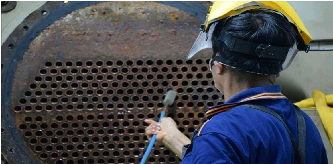
Figure I.7: Example of corrosion on a refinery distillation tray [34].
