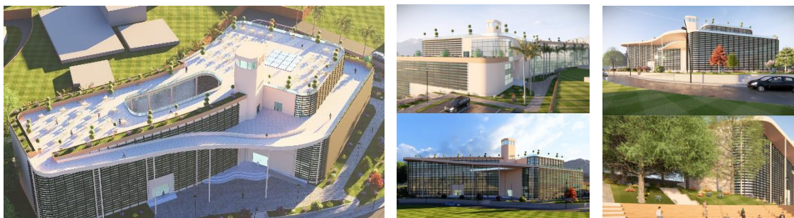
Figure 3.75: Facades of our project. Source: Authors.
