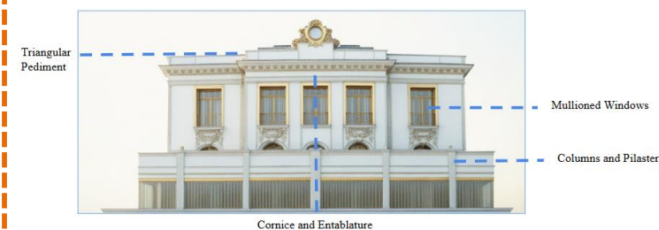
Figure 3.44: Seat of the Daira of Miliana. Source: Facade Treated by the Authors.
