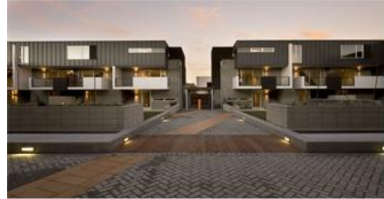
Figure 12: Photo montrant projet du Wilton Close city.
