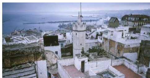
Figure 65: Terrasses de la Casbah.
