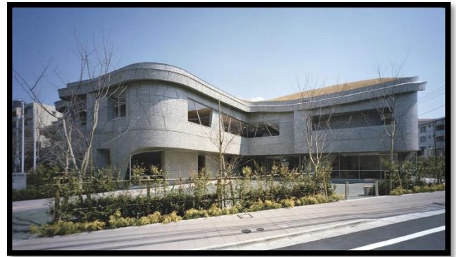
Figure 69 la façade principale de projet de KARAKIDA. Source : (Gallery of Karakida Community Center / Chiaki Arai Urban and Architecture Design - 11, n.d.)
