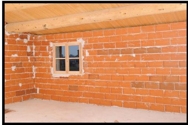
FIGURE 7 CONSTRUIRE UN DOUBLAGE EN BRIQUES SOURCE:
