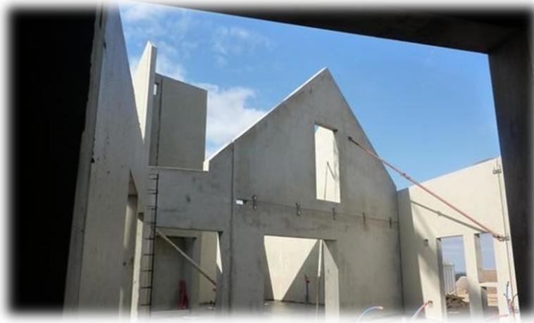
FIGURE 8 MURS PORTEURS EN BETON ARME. SOURCE: [HTTPS://WWW.BATIPRODUITS.COM/](https://www.batiproduits.com/)
