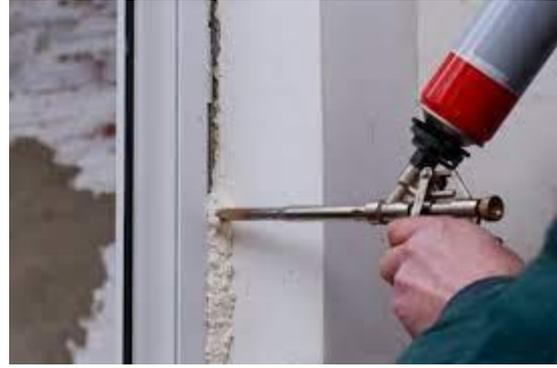
FIGURE 102 LA MOUSSE POLYURETHANE SOURCE :
