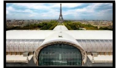
FIGURE 14 ENVELOPPE EN TEXTILE . SOURCE: [HTTPS://WWW.VERRE-MENUISERIE.COM/](https://www.verre-menuiserie.com/)
