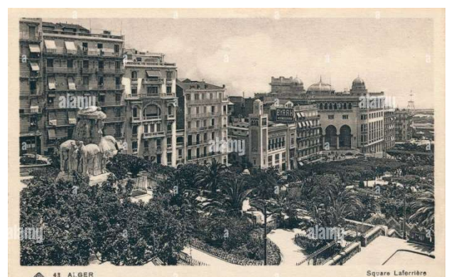
Figure 23. Square Laferrière- Alger
