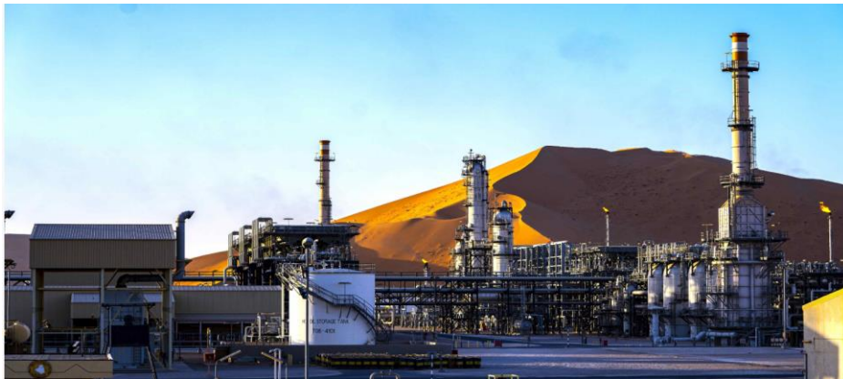
Figure 1.2: station de production [5]
