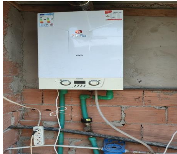
Photo 4: installation chaudière a gaz
