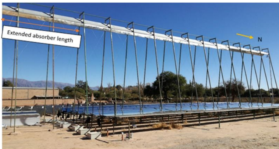
Fig.2. 15. Non-rectangular LFC prototype with southward extension in San Carlos, Argentina [144].
