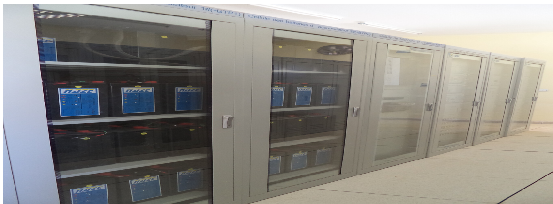
Figure 3.18: UPS power supply batteries
