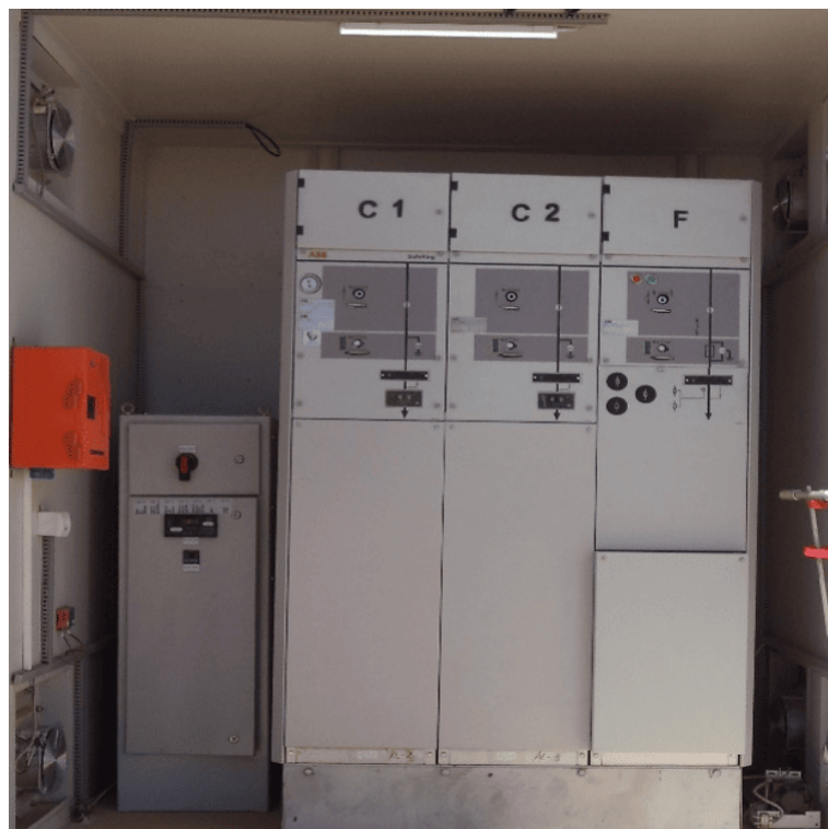
Figure 3.10: SafeRing-36kV
