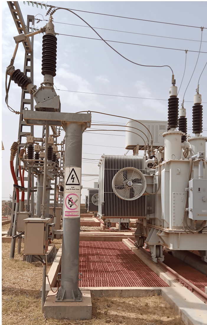
Figure 3.14: Transformer type «SFZ11-20000/60»
