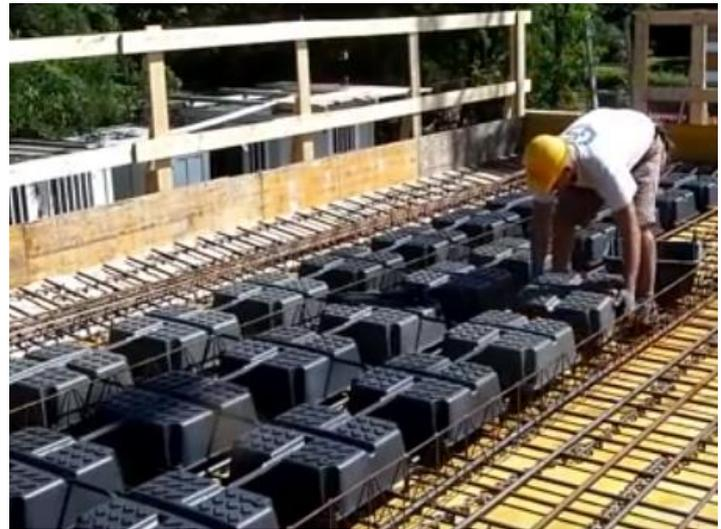
Figure 31: Plancher U-boot
