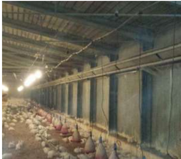
Figure 16: Mur en Panneaux sandwich
