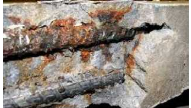
Figure 19: La corrosion
