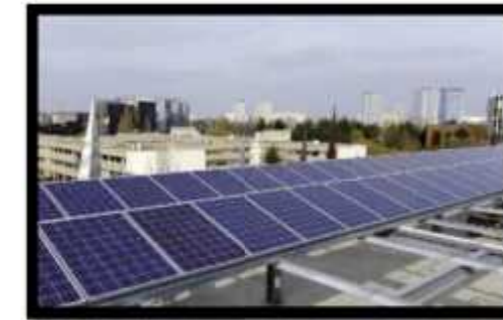
Figure 16 :les panneaux solaires source:www.iledenante.com/files/documents/pdf/publication/nante-ecoquartier.pdf
