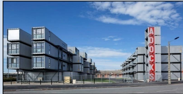
Figure 22: La residence A Dock
