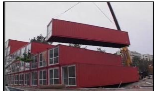
Figure 130 : assemblage conteneur
