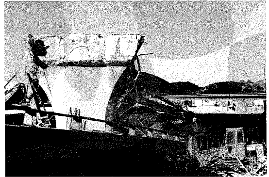
Pont 14 South Connector [11], Séisme de Northridge –Los Angeles 1994
