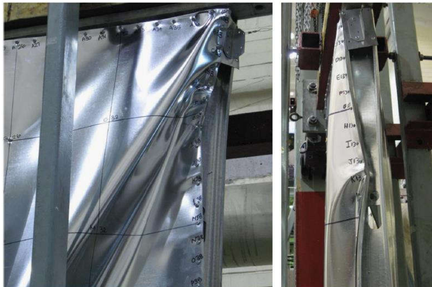
Fig. 1.12. Torsional failure of chord studs in un-blocked walls due to horizontal component of tension field force, at left: face view of 1220 x 2440 mm SWP (monotonic loading) and at right: end view of 610 x 2440 mm SWP (monotonic loading) [17].
