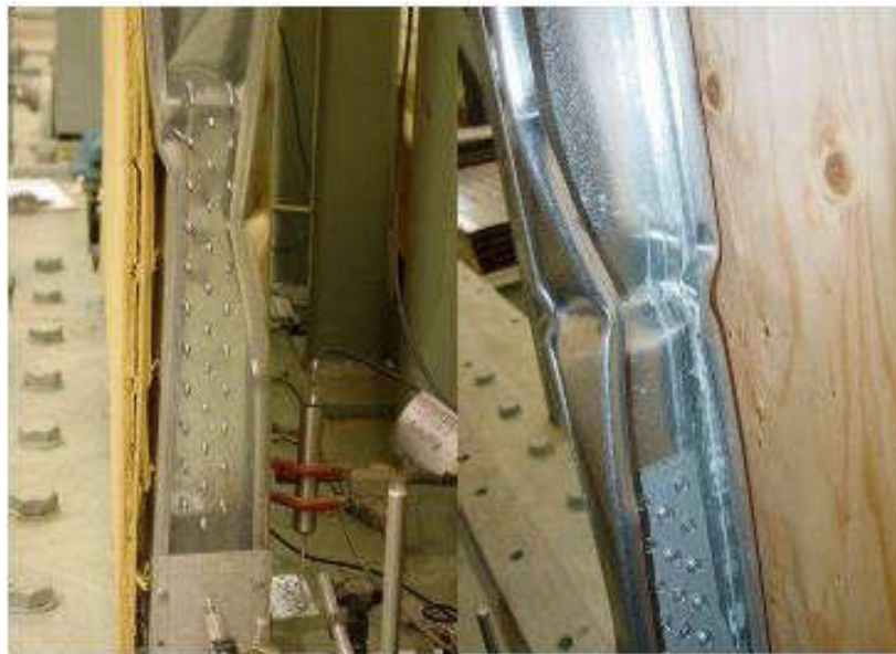
Fig. 1.16. Local buckling of the chord stud [11].
