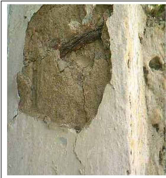
(c) Ouvrage prive, Boufarik
