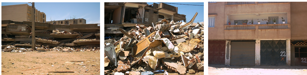
Figure 5. Damage contrast in adjacent buildings
