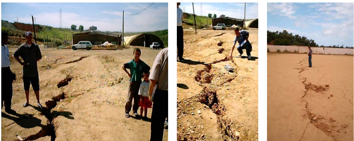
Figure 1.11 : Fissurations des routes
